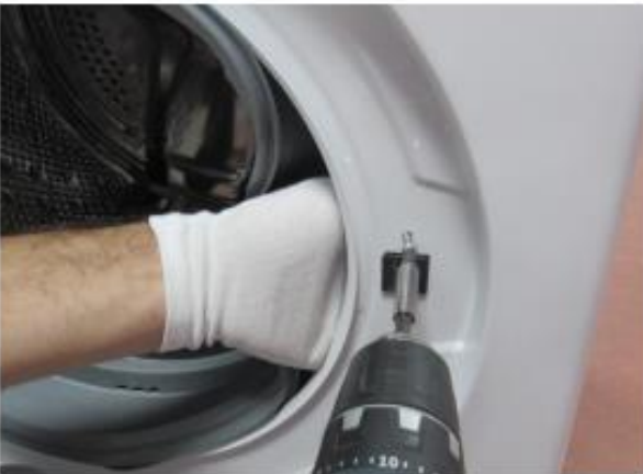
Tighten the door lock screw
