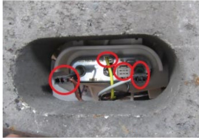
Remove the heater sockets
