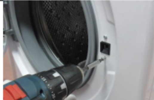
2.6. Remove the screws fixing the door lock.
