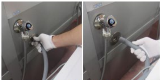
Disconnect the drain hose
