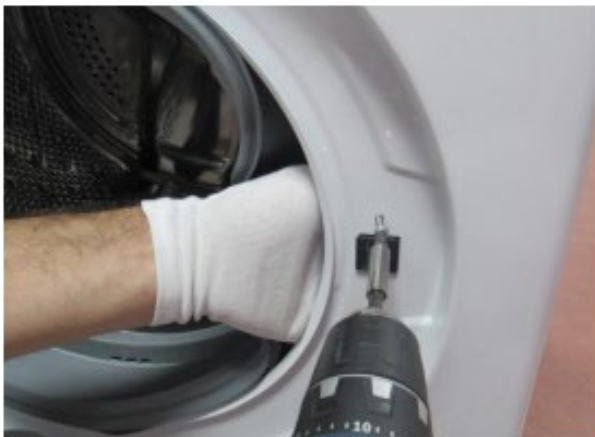
Tighten the door lock screw
